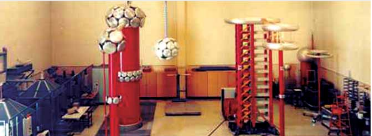
High Voltage laboratory
