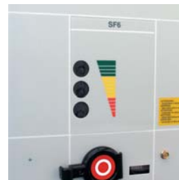
SF6 control device with 3 LEDs.
